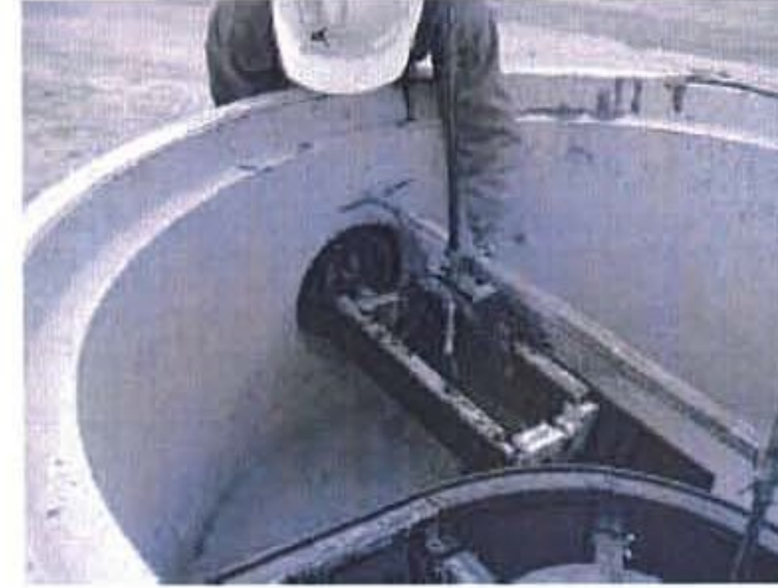
#4 POSITION ANTI FLOTATION BAR AND ADDITIONAL CHANNEL
