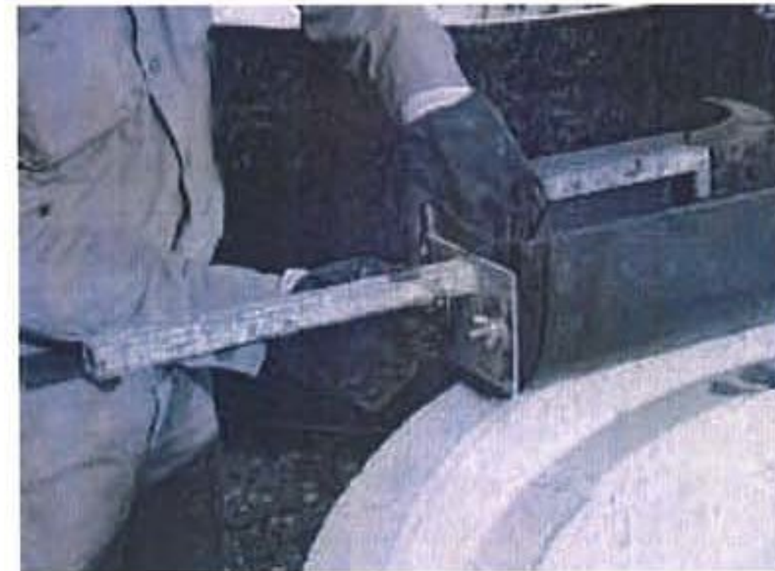
#2 ASSEMBLE SMALLEST ANGLE WITH CENTERING ADAPTOR
