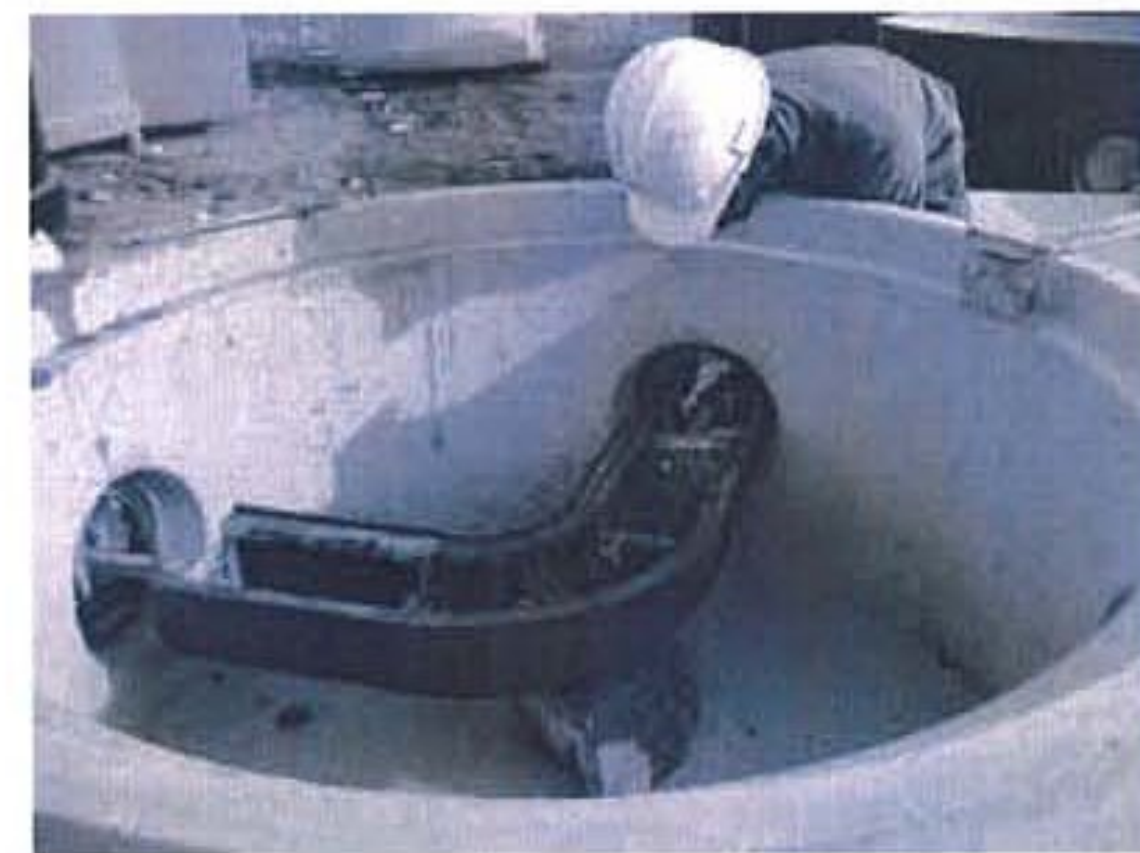
#3 SMALLEST ANGLE ASSEMBLY IN LOW HOLE AND UPSTREAM SIDE.
