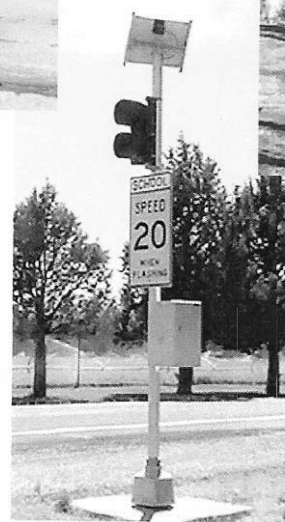
Typical Solar Powered System
