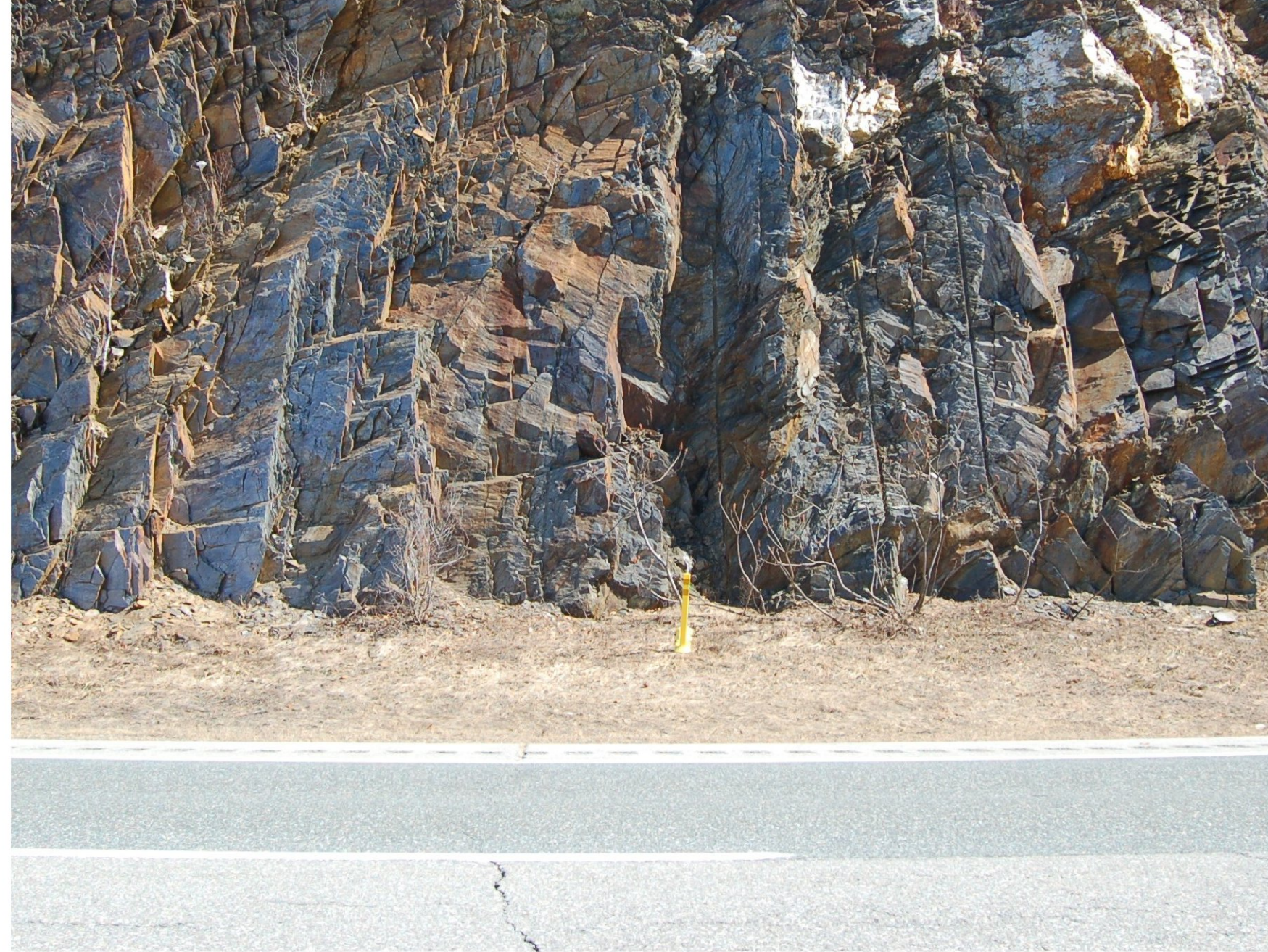
STA. 1857+50 MACHINE SCALING AT TOP ONLY
