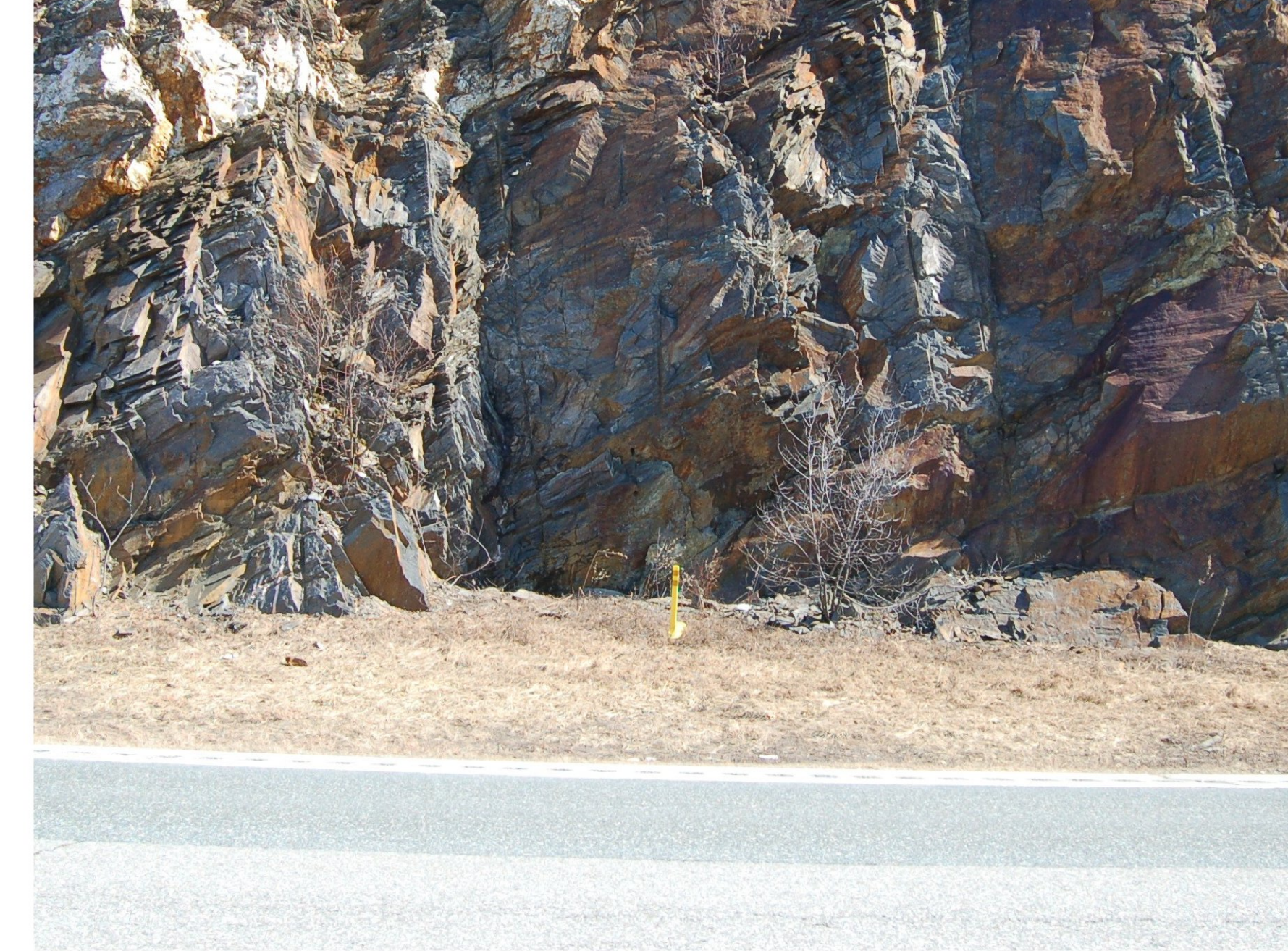
STA. 1857+00 MACHINE SCALING AT TOP ONLY
