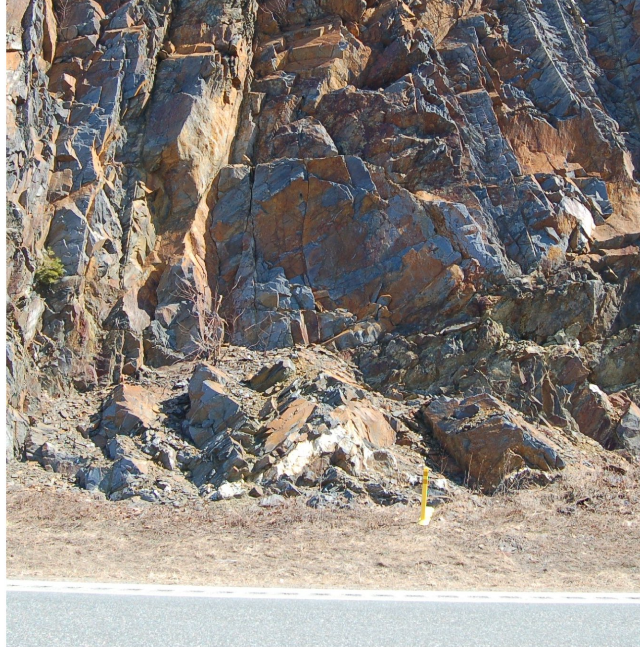
STA. 1855+50 MACHINE SCALING AT TOP ONLY
