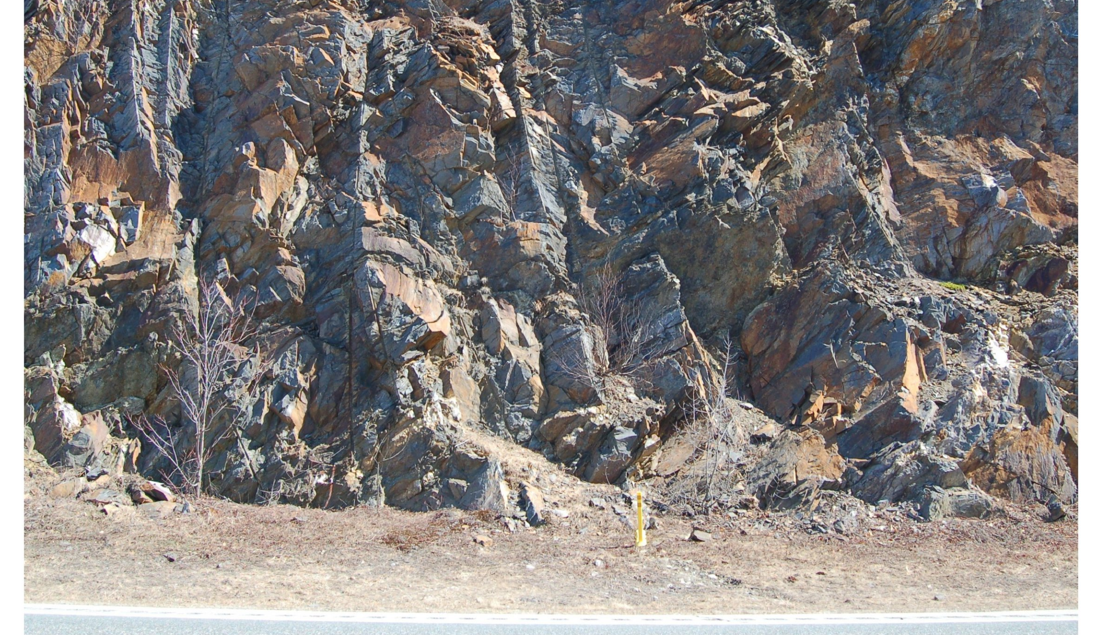
STA. 1855+00 MACHINE SCALING AT TOP ONLY
