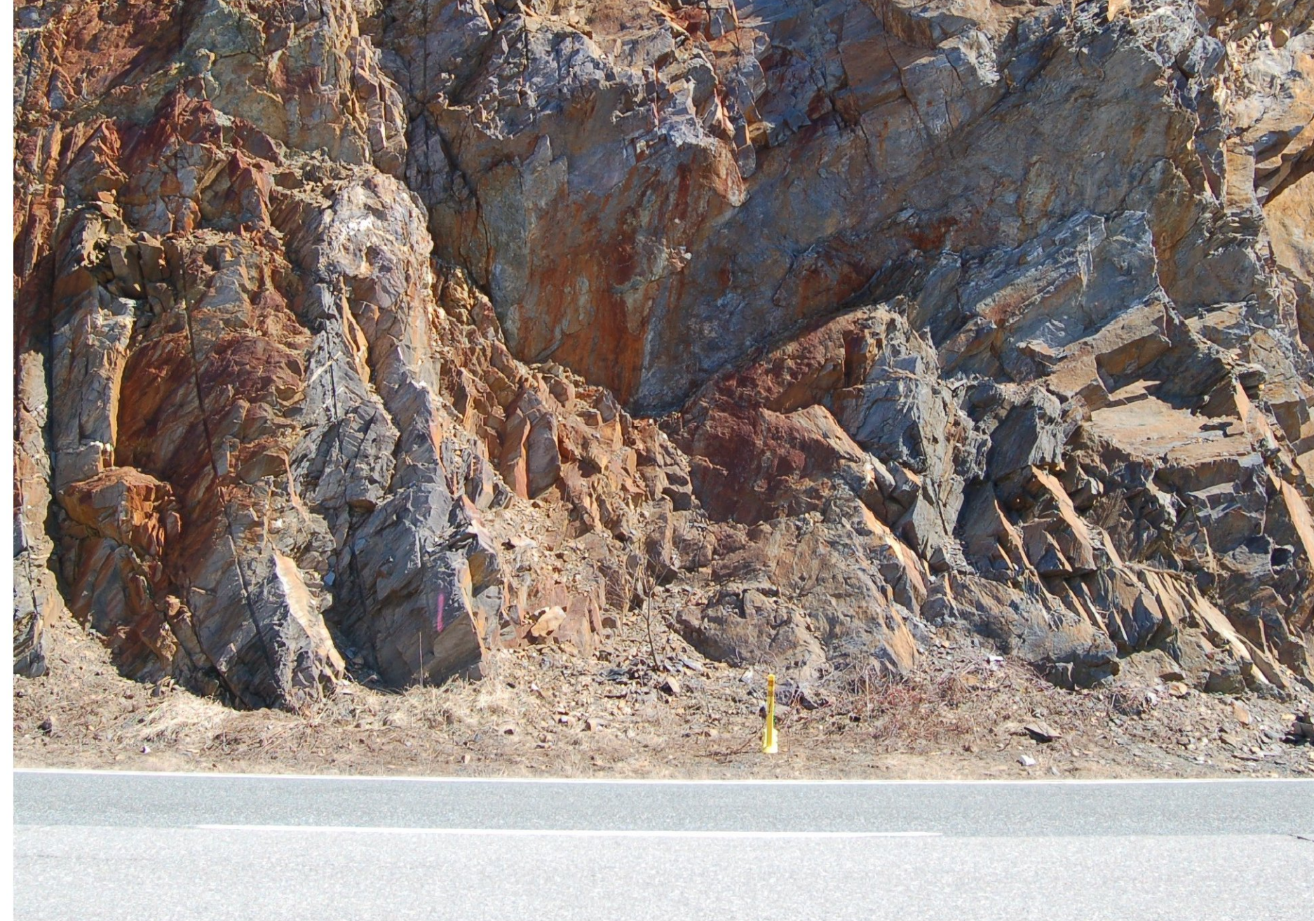
STA. 1853+50 MACHINE SCALING AT TOP ONLY
