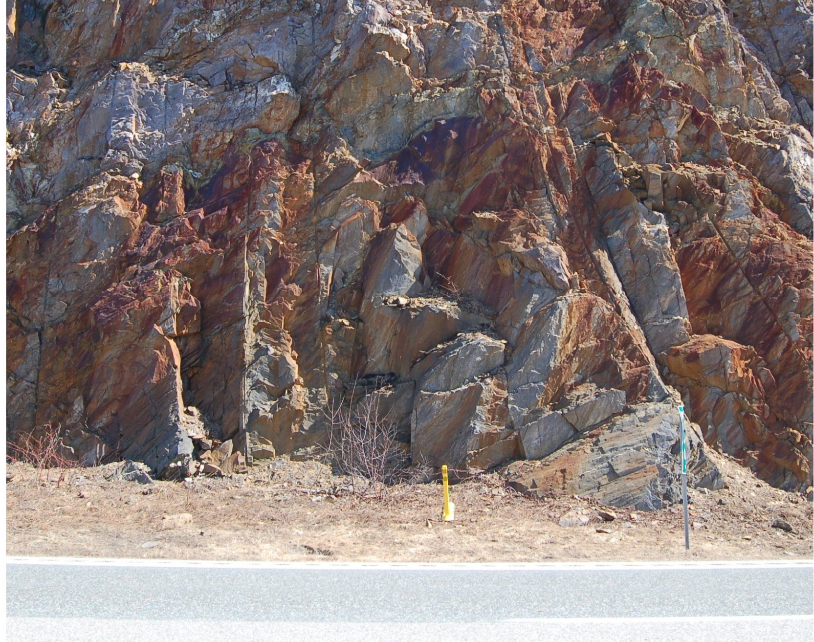
STA. 1854+00 MACHINE SCALING AT TOP ONLY
