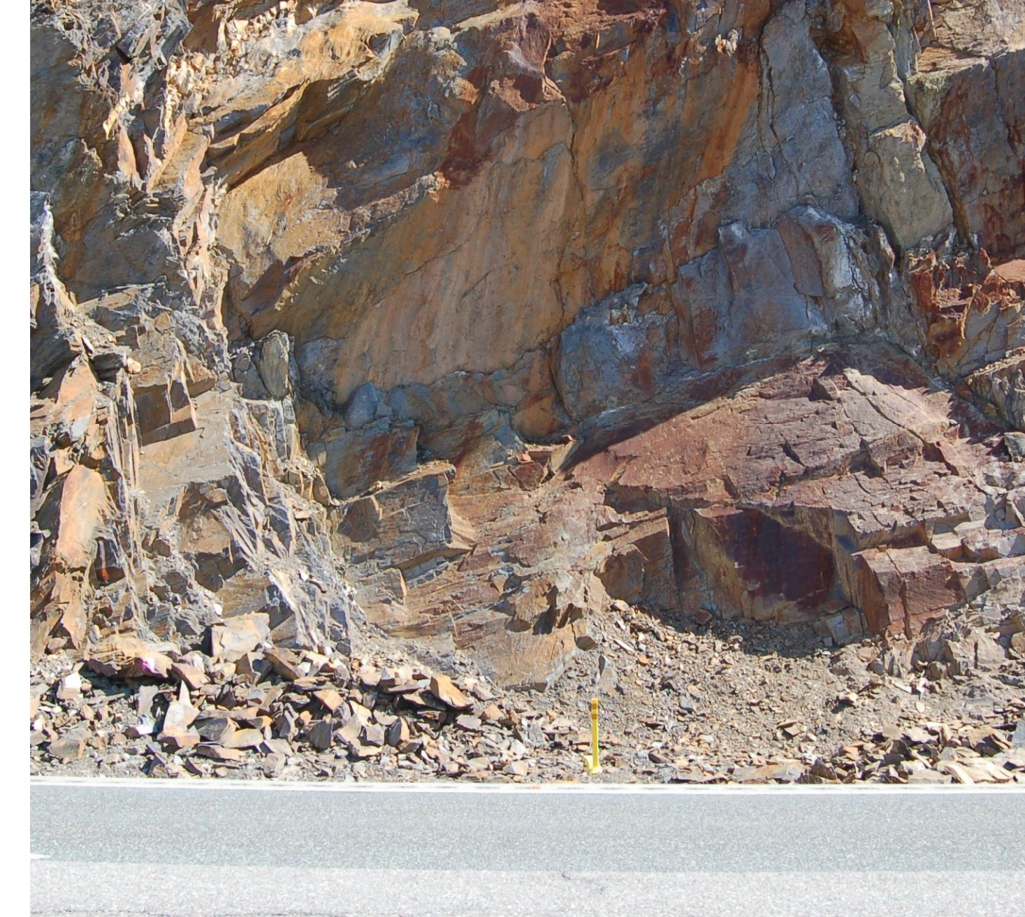
STA. 1853+00 MACHINE SCALING AT TOP ONLY
