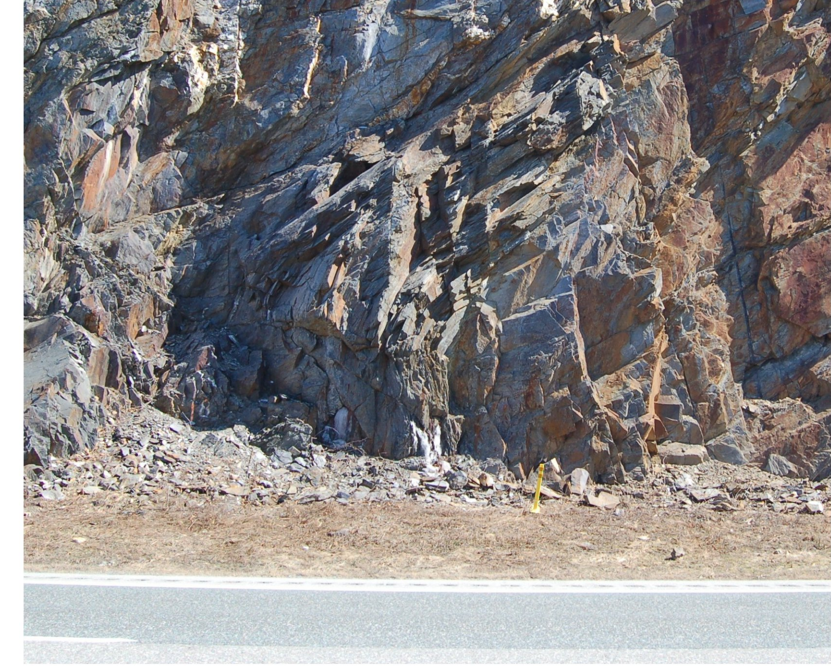
STA. 1851+00 MACHINE SCALING AT TOP ONLY
