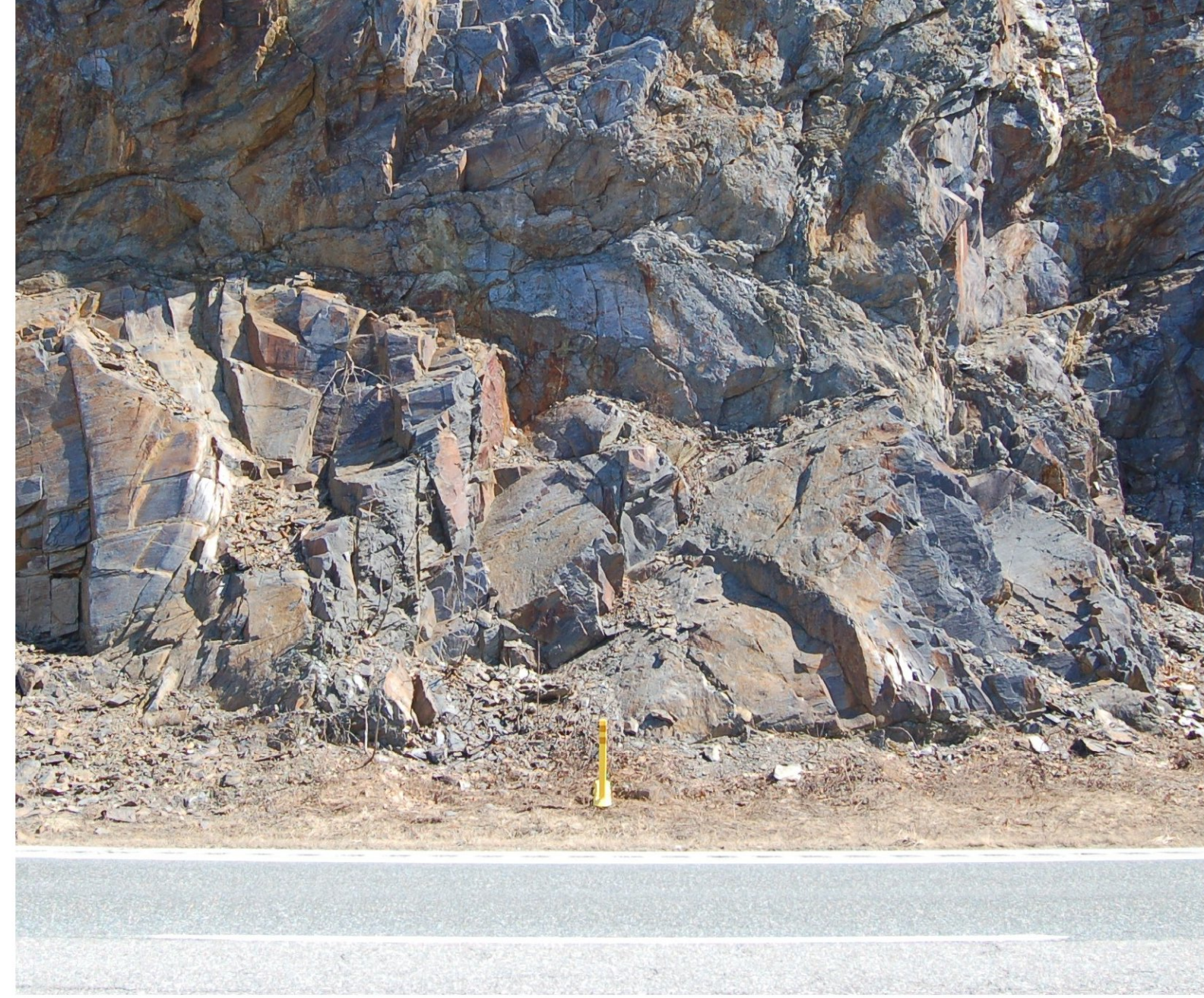
STA. 1851+50 MACHINE SCALING AT TOP ONLY
