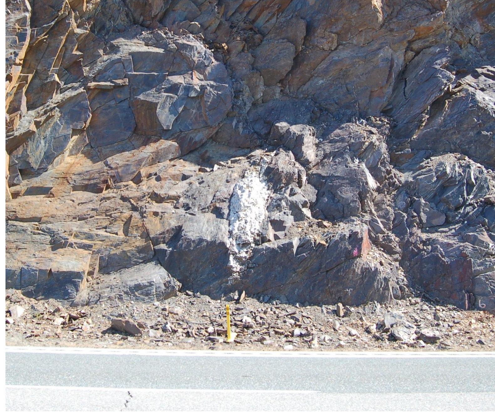
STA. 1849+50 MACHINE SCALING AT TOP ONLY
