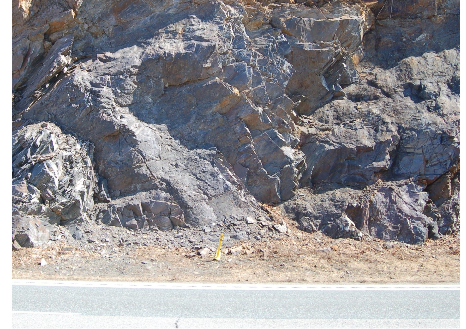
STA. 1849+00 MACHINE SCALING AT TOP ONLY
