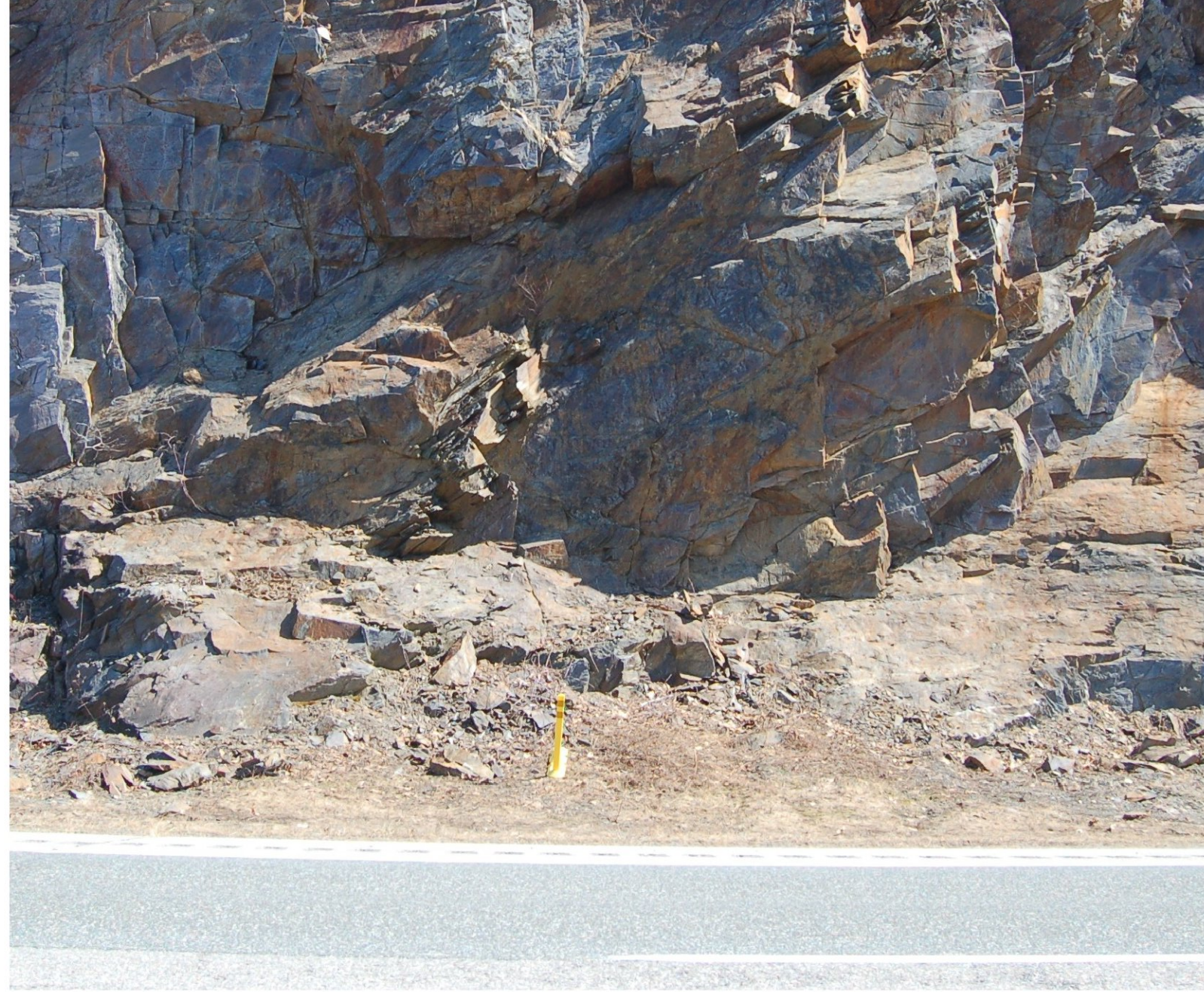
STA. 1850+00 MACHINE SCALING AT TOP ONLY
