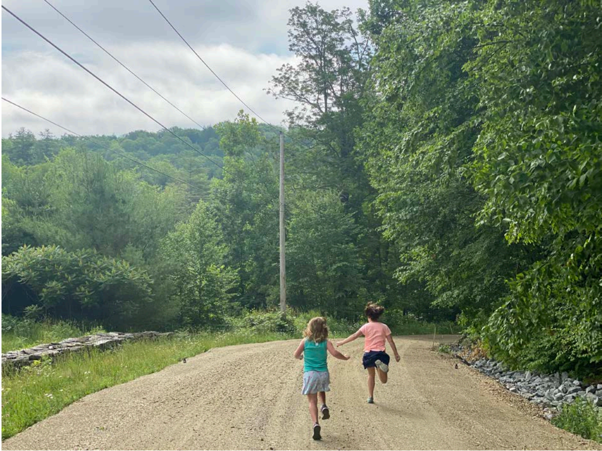
New portion of Gaskill Road (stone lined ditches, 22 feet width)
