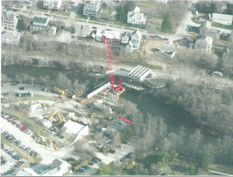
Bridge - under construction
