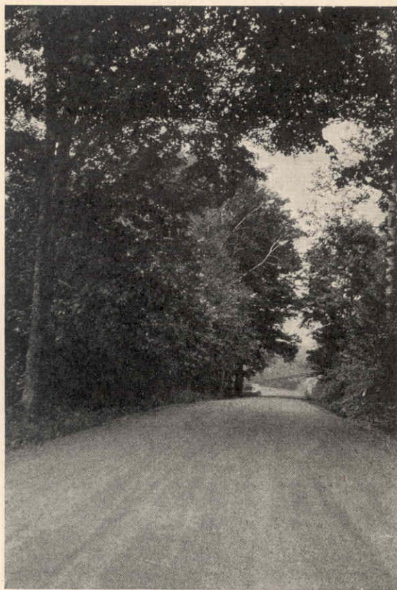
The Brattleboro-Wilmington Road, a Federal-aid gravel road constructed in 1920. The photograph shows the excellent condition of the surface in 1924
