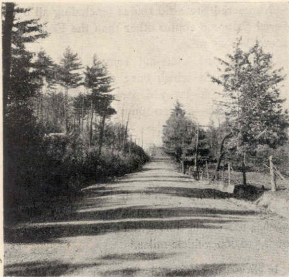
Federal-aid Project No. 13, near Addison, a bituminous macadam road
