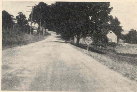
U. S. Route No. 5, near Hartland. The road is surfaced with gravel. Note the standard caution sign
