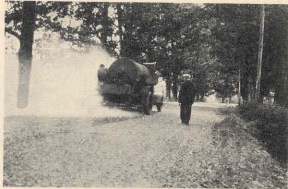
Applying seal coat on the Bernardstown Road
