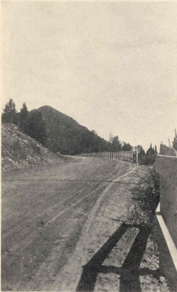
The Molley's Brook Road—A gravel road treated with calcium chloride
