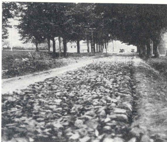
A stone base under construction north of St. Albans
